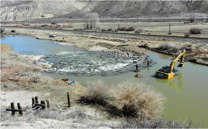
The LCD sponsored the replacement of a large irrigation water diversion structure on the Bear River north of Cokeville, WY.
