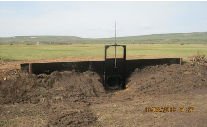
One project completed this past year was an irrigation water control structure in the Upper Hams Fork River Watershed by the NRCS for a district cooperator.
